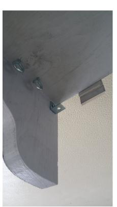
11. Tie cord onto the bottom ring of blind, thread it through the rings going up the blind, and into the screw eye mounted on the bottom of the poplar. Bring the left side cord across and thread it through the right side screw eye mounted on the bottom of the poplar, so that both cords are now together.
