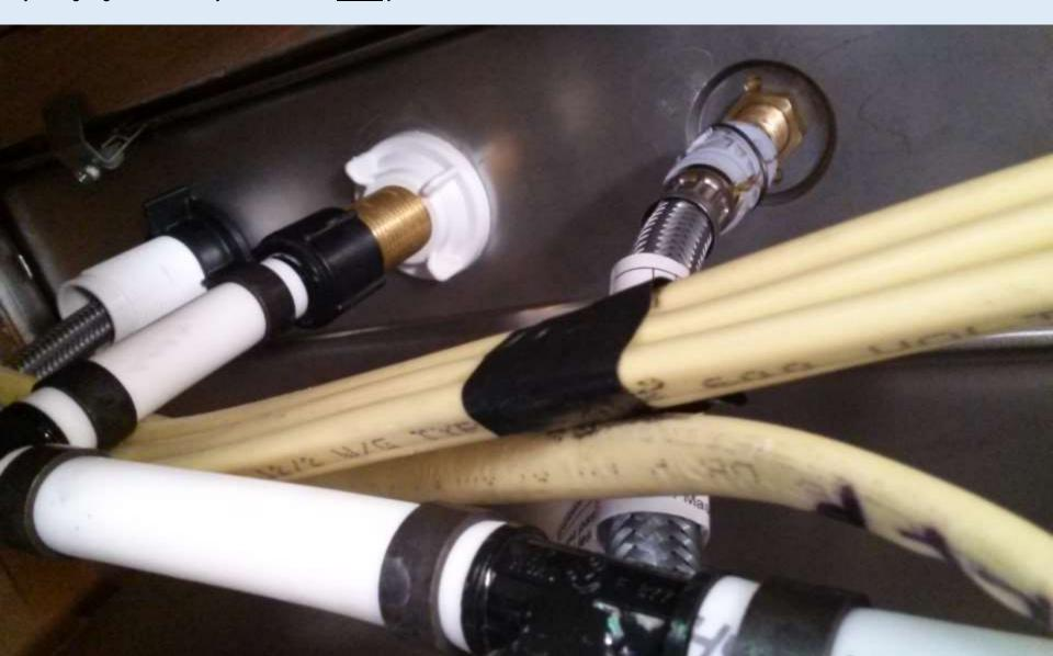
Once you are satisfied that you have no leaks, shut of the water supply to the trailer, and relieve pressure to the system by opening the drain valve in front of the driver's side tire on the outside of the trailer, and both faucet valves. Then remove the water heater bypass line, and reinstall the water heater (see the separate tutorial). Finally, pat yourself on the back. You've got a new kitchen faucet that not only looks nice, but also allows you to buy repair parts in the future.
