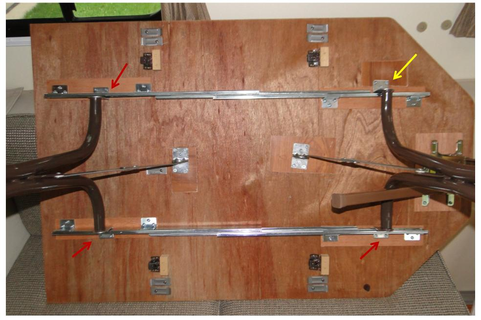
Close up showing leg secured under the leaf sliding mechanism.
