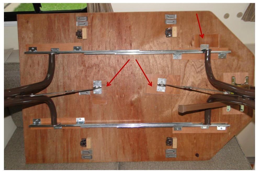
Three of the four legs were able to be secured underneath the sliding table leaf mechanism (red arrows). One side would easily slide underneath, then the other side I had to remove the screws of the fastener, and then slide the leg under. The fourth one (yellow arrow) had to be secured on the outside of the mechanism, thus requiring a thin piece of wood to match the height.
