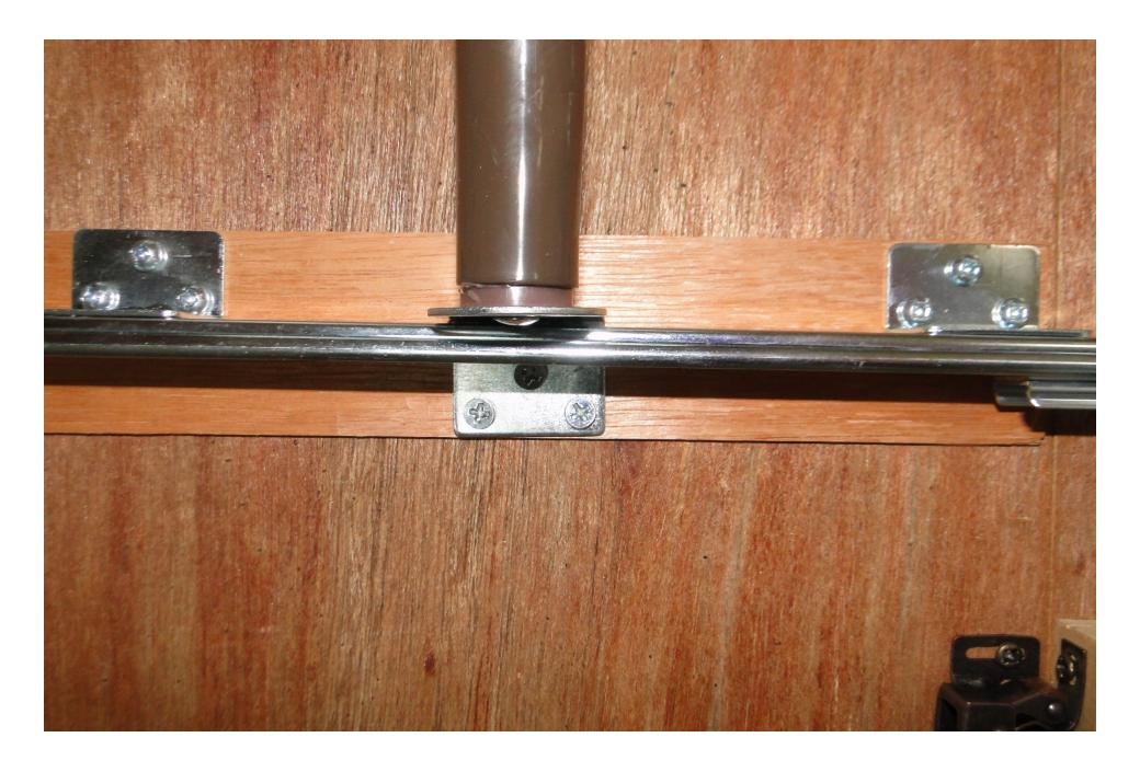
Close up showing 4<sup>th</sup> leg secured over the top of the leaf sliding mechanism.
