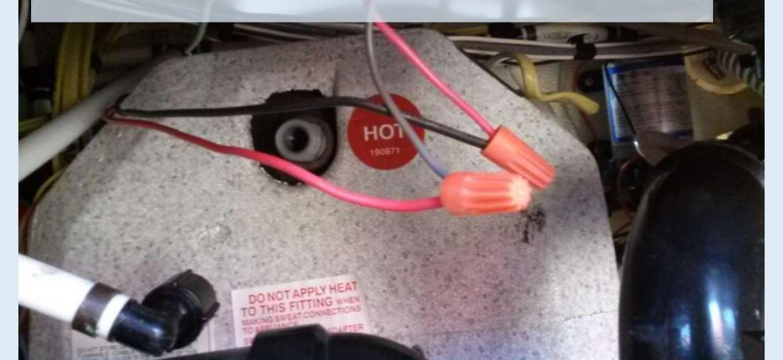
9. Disconnect the three 12vdc wires that go the systems monitor panel. You will probably find that the negative/neutral wire (green) is not connected by wire nut. I advise cutting this wire and reinstalling it with a wire nut, as shown. You will probably have to cut a zip-tie to bring these wires down in order to work on them, as I have done here.
