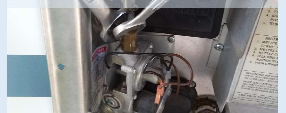
6. Open the propane tanks on the trailer to pressurize the gas lines. Apply a soapy solution (dish soap and water) around the fitting to check for leaks. (The bubbles you see here do not represent a leak; they are just "foam." A leak will create much larger bubbles.)
