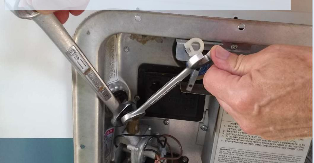
8. Go inside the trailer, and disconnect the water supply lines from the back of the water heater. It's helpful to have an old towel to catch any drips.
