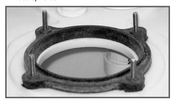
16. Place toilet on studs and secure with four washers and four nuts.
