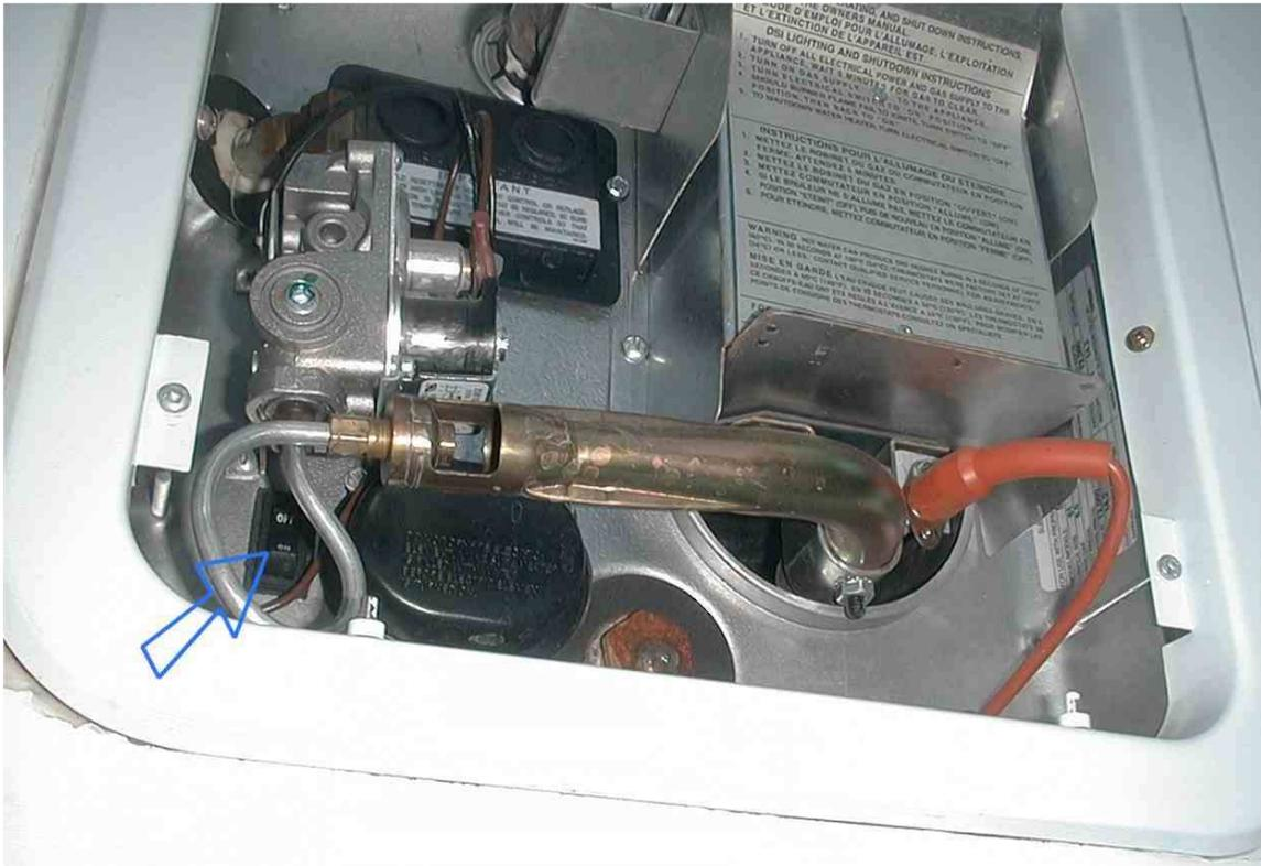
**THE CARDINAL RULE OF WATER HEATERS:** You must always make sure that the water heater is full of water before you turn on either heating element. If you dry fire it on gas, you probably have a few seconds, no more, to correct your mistake. If you dry fire it on electric, even for a moment, the electric element will probably burn up. It is not hard or expensive to replace the element, but it is always inconvenient.
