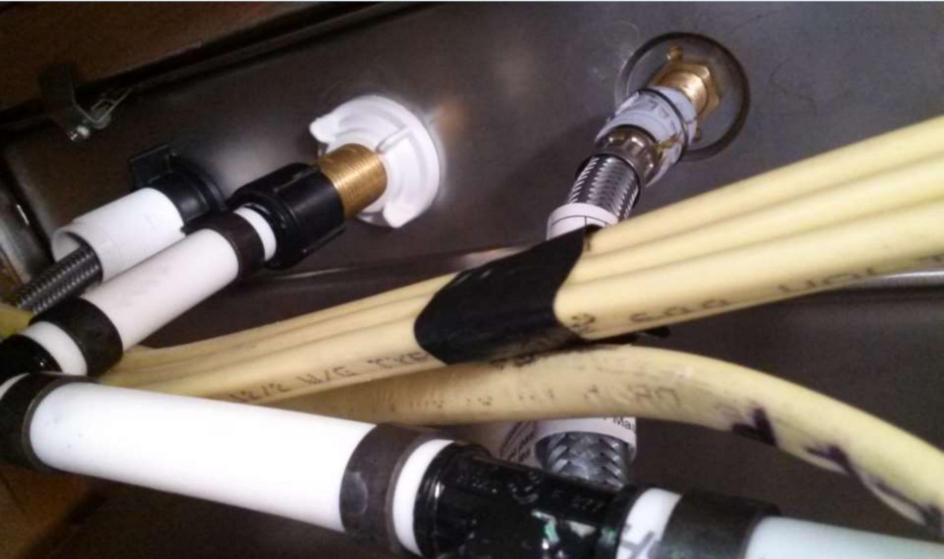
Once you are satisfied that you have no leaks, shut of the water supply to the trailer, and relieve pressure to the system by opening the drain valve in front of the driver's side tire on the outside of the trailer, and both faucet valves. Then remove the water heater bypass line, and reinstall the water heater (see the separate tutorial). Finally, pat yourself on the back. You've got a new kitchen faucet that not only looks nice, but also allows you to buy repair parts in the future.
