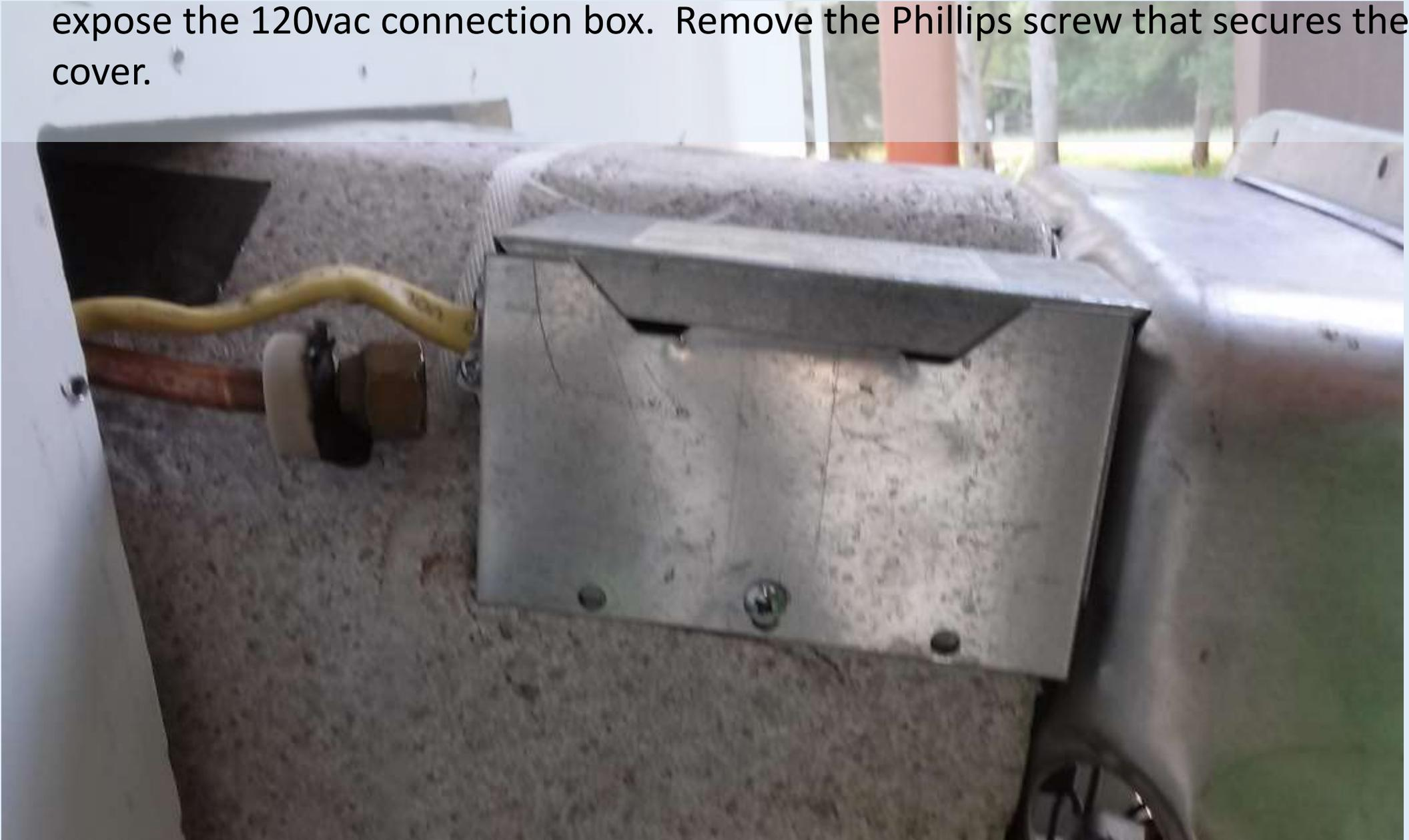
15. Remembering that the first step was to disconnect shore power, disconnect all three leads, and loosen the cable clamp (arrow) so that the cable can be pulled free of the WH.
